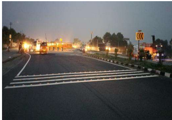
Road Diversion in the night
